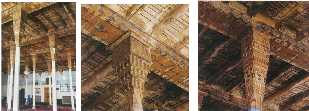
Fig.21a,b,c. Chamber(Shabestan) of Mehr- abad mosque; Sample of capitals in Mehr- abad mosque- Bonab
