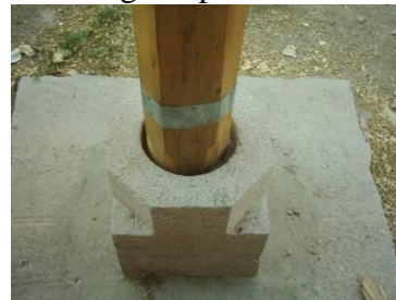
Fig. 24b: Restored foundation and stone base
