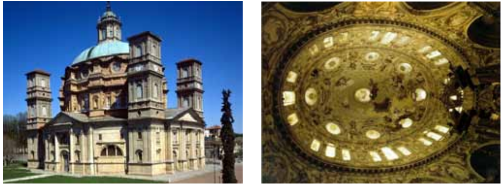
Fig. 2. (left) External view of the Basilica and (right) the interior of the dome.
